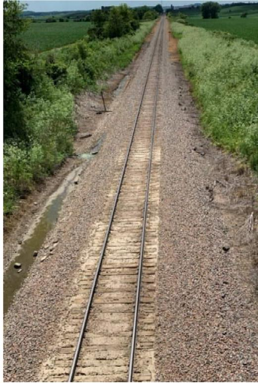
**Figure 16: Photo taken from the E Roberts Rd Crossing depicting track with fouled ballast and a ditch with standing water**
