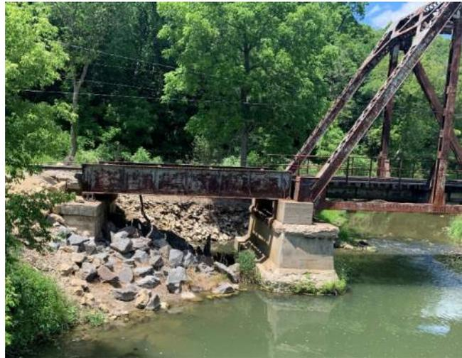
**Figure 19 & Figure 20: One of several bridges of the East Fork Galena River east of Galena. Deterioration of the concrete pier and rusting of the steel members is visible.**
