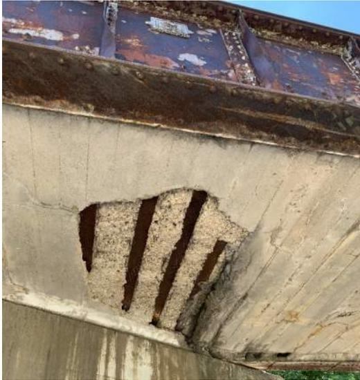
**Figure 17: E Yellow Creek Rd crossing – East of Freeport. Concrete spalling and rusting of the steel girder is evident.**
